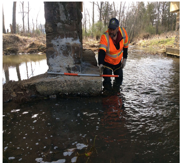
PHOTO 2 Description Undermining to inlet end of Bent #4, photo #2.
