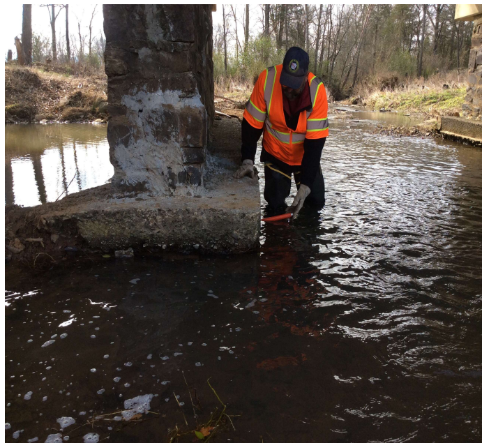
PHOTO 1 Description Undermining to inlet end of Bent #4, photo #1.
