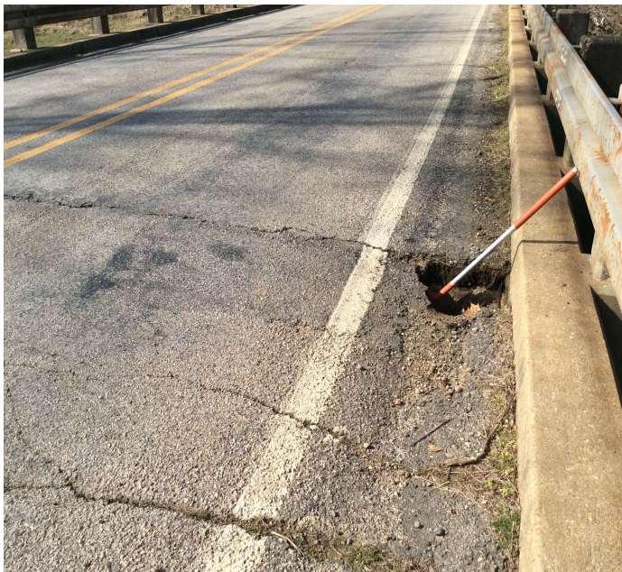
PHOTO 1 Description Settlement at East approach.
