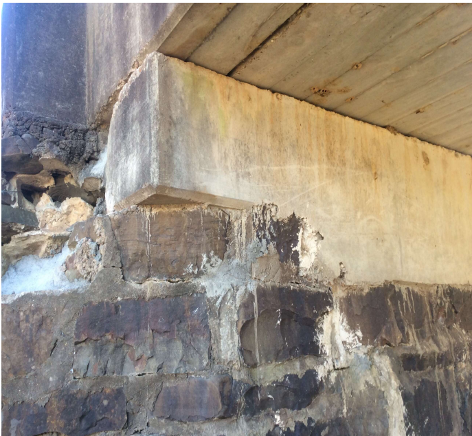
PHOTO 1 Description Rock missing behind the cap at Bent # 5 left side.
