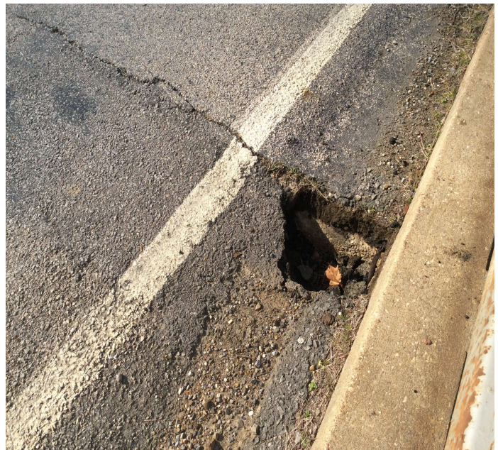
PHOTO 2 Description Settlement in the East approach roadway with a hole in the Left shoulder at the bridge end.
